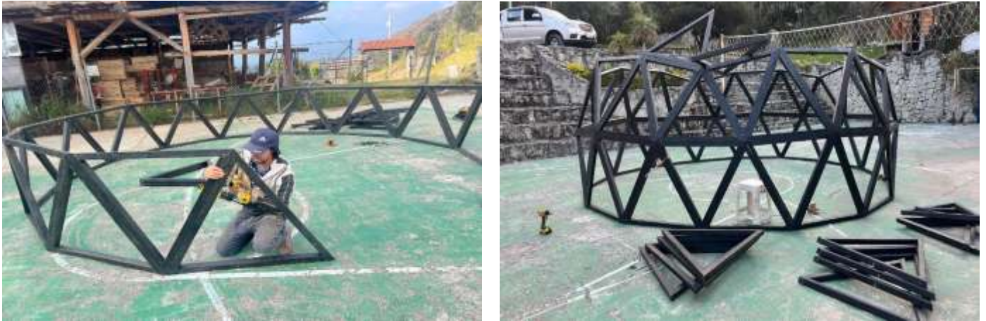
Figure 17 Assembly of the first strip and Dome at 50% completion.
