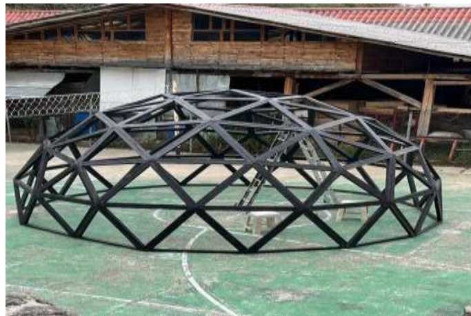
Figure 18 Geodesic dome with recycled polypropylene plastic elements.
