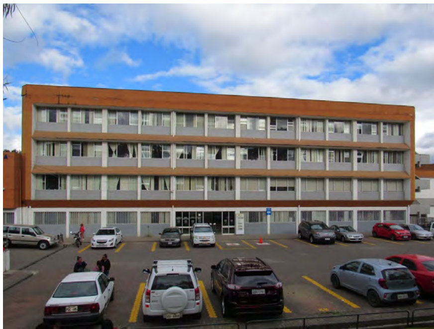
FIGURA 2.59: Fachada principal, Hospital Homero Castanier Crespo
