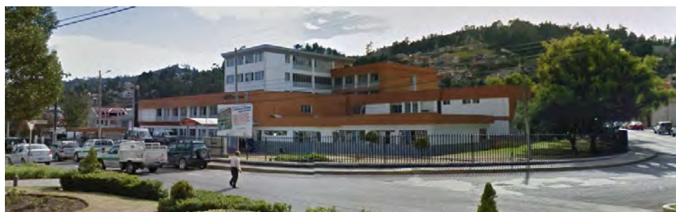
FIGURA 2.40: Cerramiento Hospital Homero Castanier Crespo
