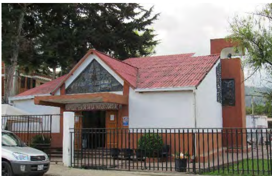
(a) Fachada principal
