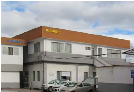
(a) Fachada principal
