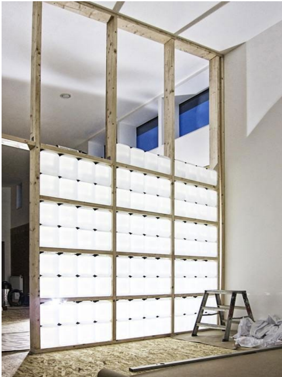
Figura 67: Muros internos Upcycled House
